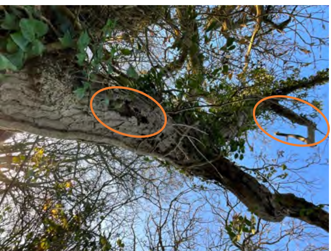
T28 – Lifting bark and stag with cavity at base
